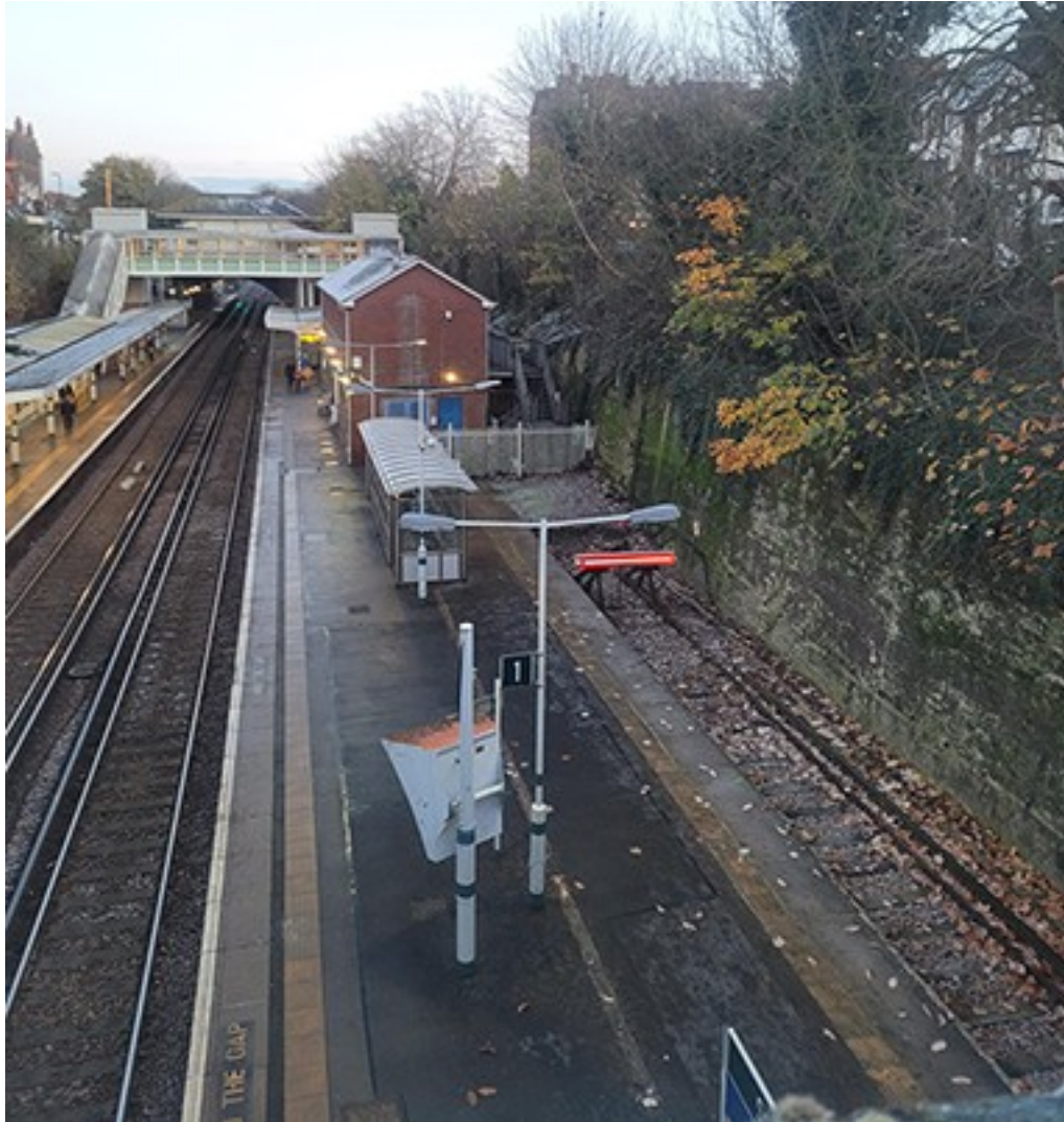
View of Streatham Hill Station from the B221 road bridge
